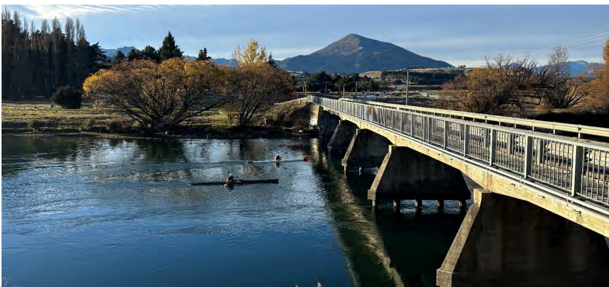
Figure 1 Kayakers Passing Under Albert Town Bridge
