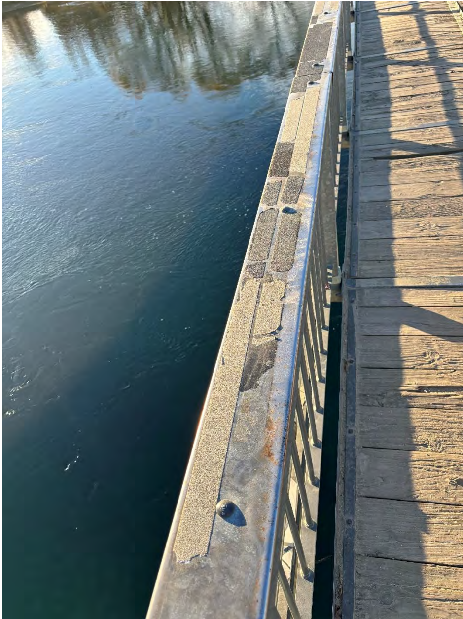
Figure 8 Grip Tape Installed on Preferred Jumping Zone
