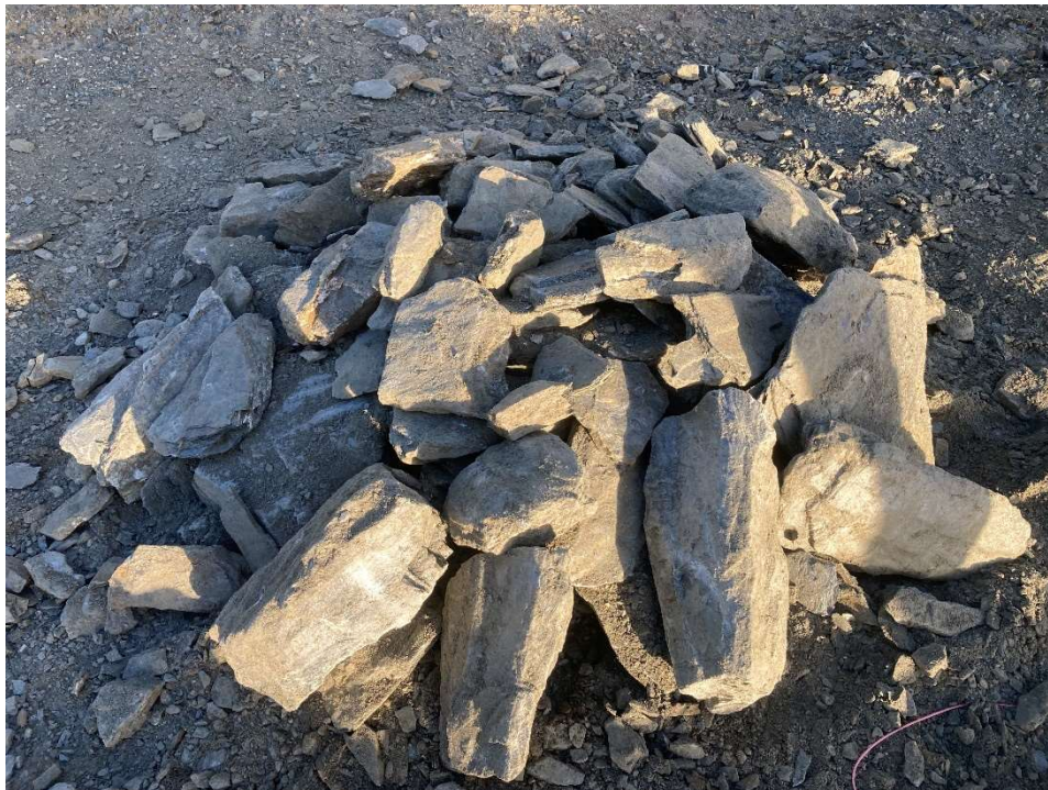
Photograph 4: Site won rip-rap to be used for lining water table drainage ditch (once reduced was appropriate)
