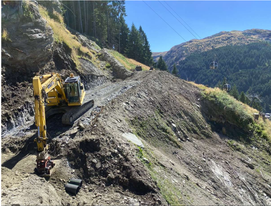
Photograph 3: Progress of culvert installation
