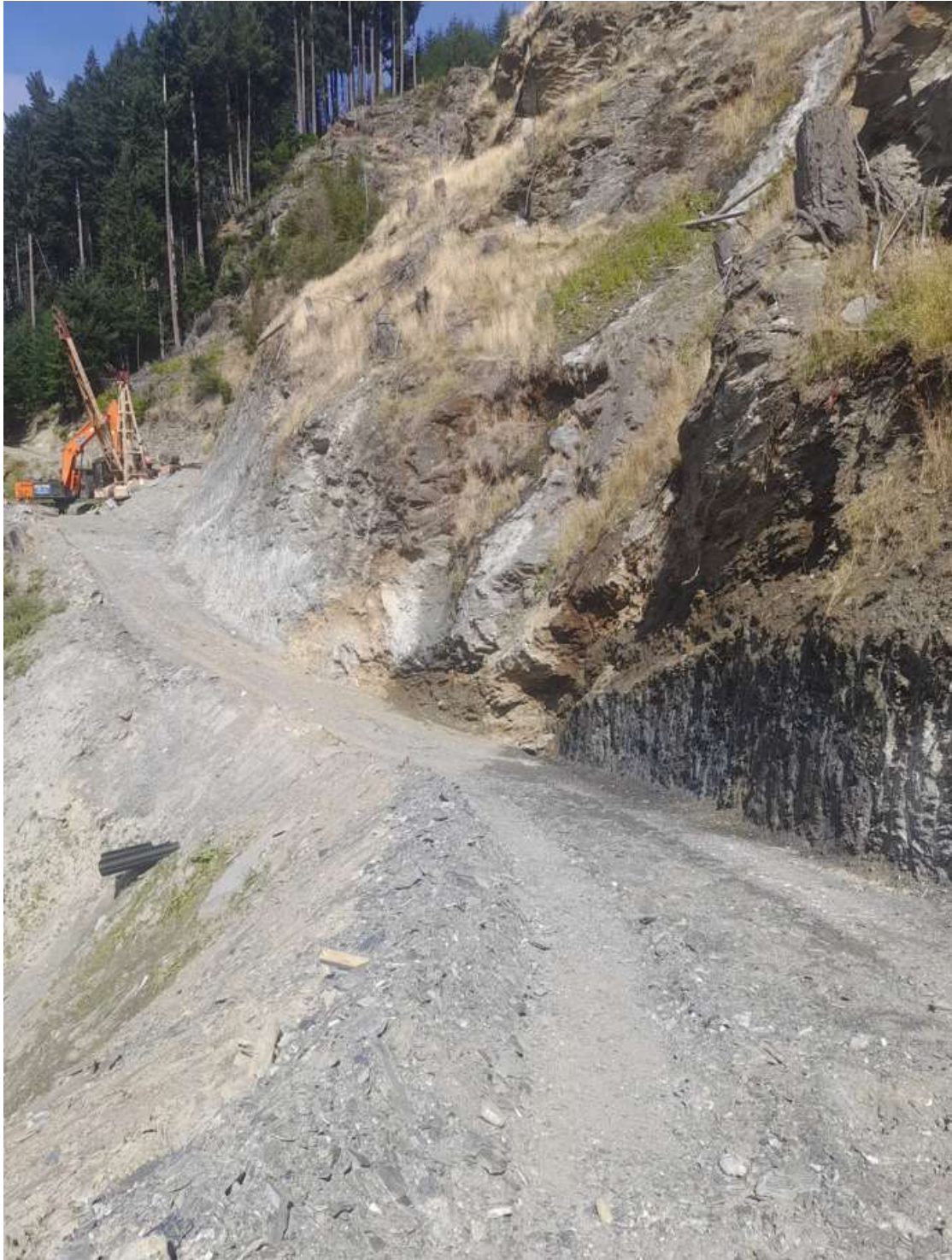
Photograph 5:- Northern Ramp showing underlying schist bedrock and upslope cut batter.
