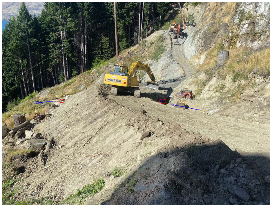
Photograph 2:- Fill batter of northwestern ramp and culvert intake/outlet and flow direction
