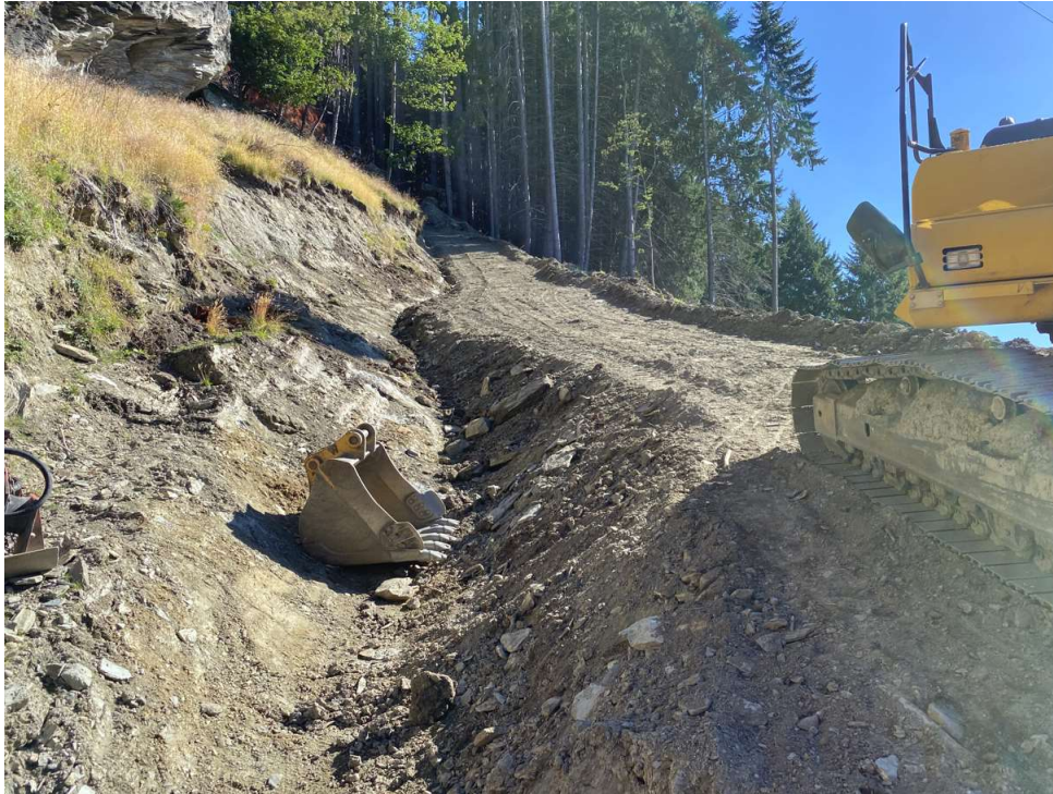
Photograph 3: Water table and upslope track cut batter
