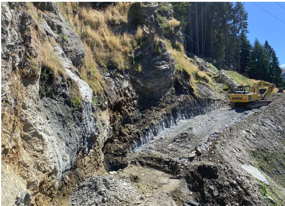
Photograph 4: Northern Ramp showing underlying schist bedrock and upslope cut batter.
