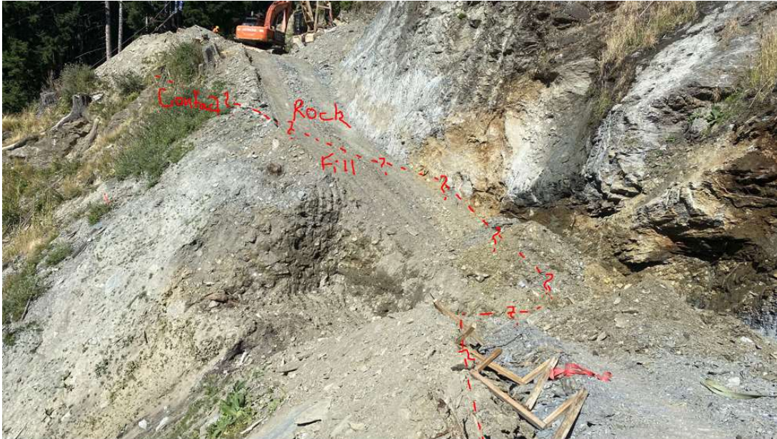
Photograph 1:- Inferred rock contact on track surface.
