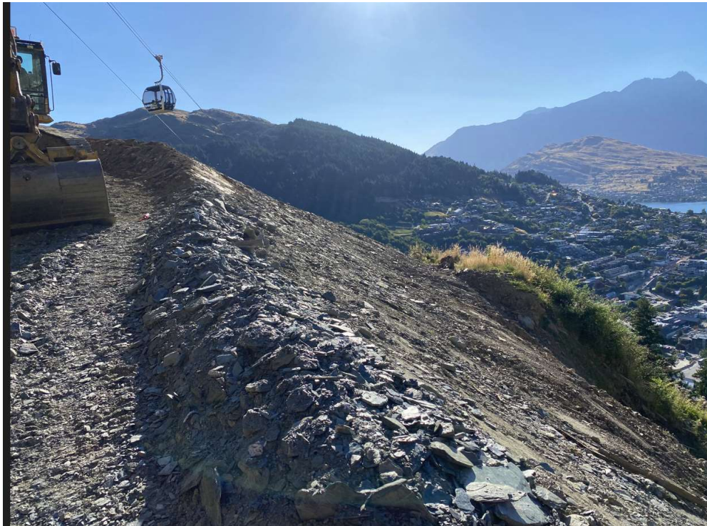
Photograph 1:- Fill batter of northwestern ramp
