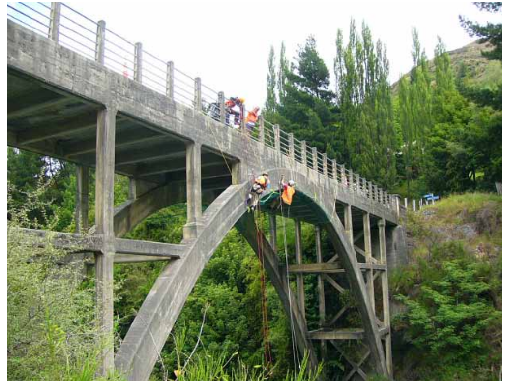
Inspecting Edith Cavell Bridge, Arthur's Point
