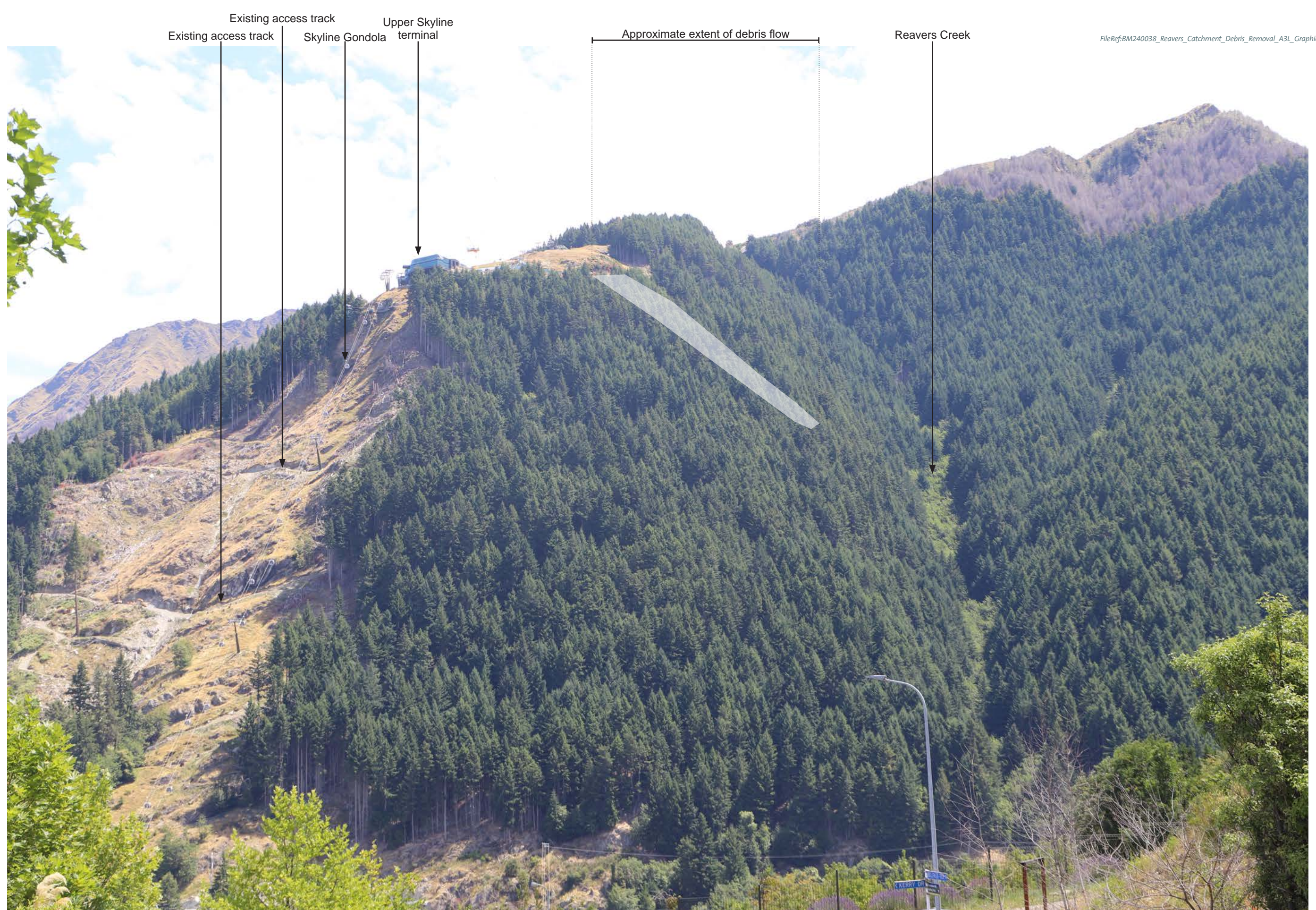
Site Context Photograph 8: Photograph taken from the start of Queenstown Hill walking track on Belfast Terrace looking in a northwesterly direction, approximately 920 metres east of the Site. Skyline Gondola and upper Skyline terminal are largely visible from this viewpoint.
