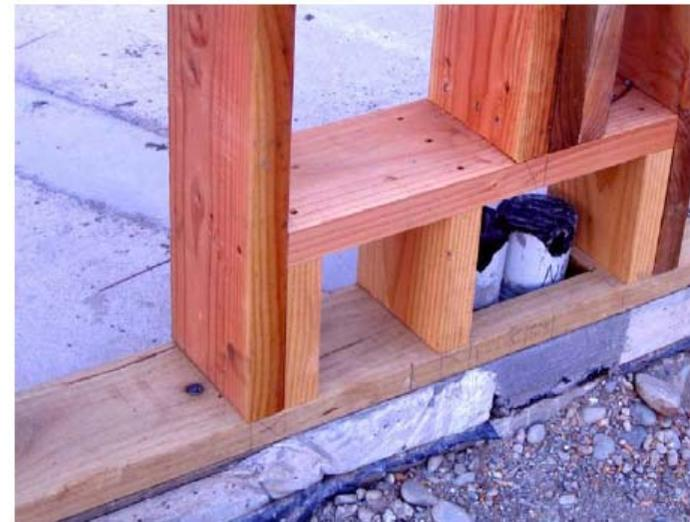
*Untreated Douglas Fir used as framing. In this case treated Radiata is used for the bottom plate.*
