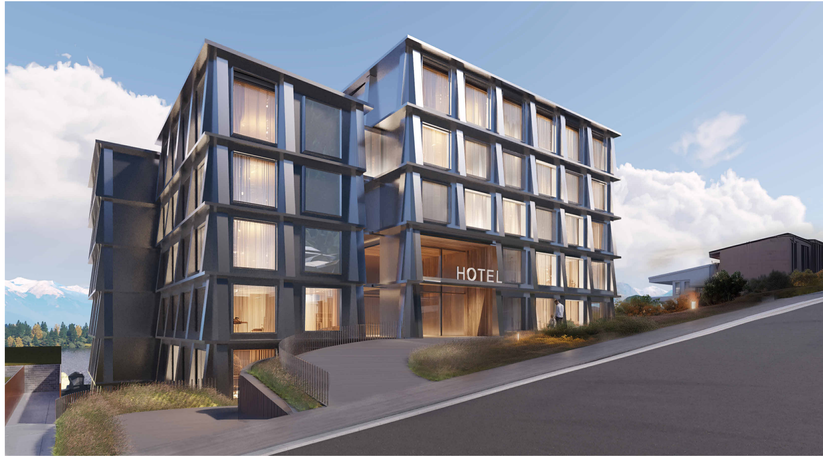
APPROACH ALONG MAN STREET
