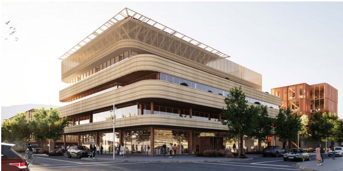
Figure 11 - View of hospital complex from Grace Wright Drive (by Warren Mahoney)
