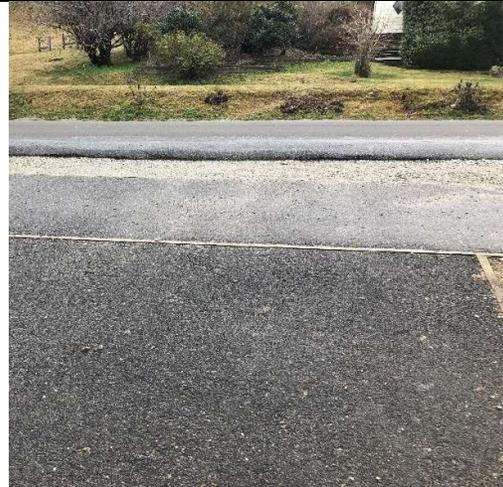
Entrance off Hedditch Street. Note, lower level and unfinished section between high road and pedestrian path. Gravel and water flow across and down here.
