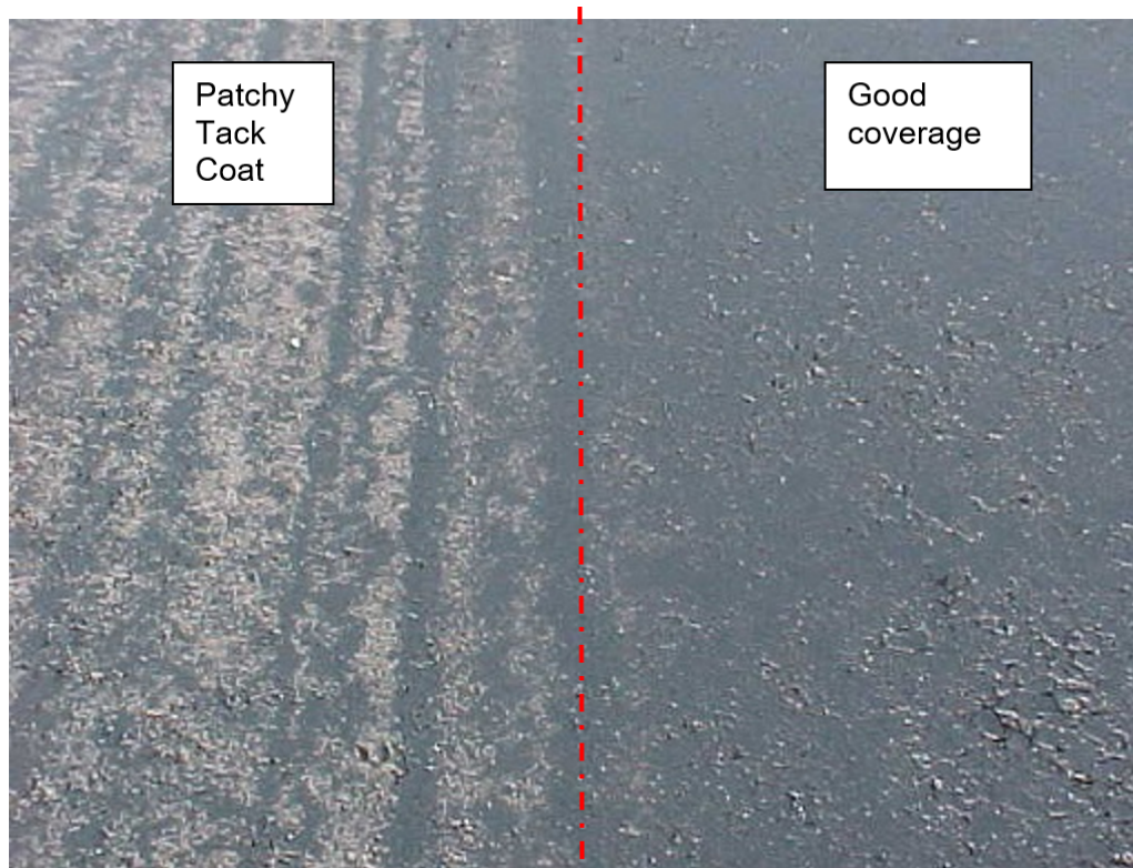
Figure 4 Tack Coat Application Examples
