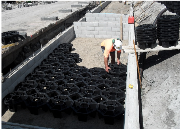
Integration of trees and infrastructure. Example of soil cells being laid out into tree pit areas. Image courtesy of Paul Malcolm, MetroGreen.
