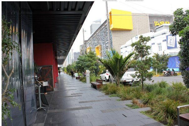
Good species selection in line with the proximity of the building. As the trees develop, some pruning required, for buildings and power line for proposed tram network.
