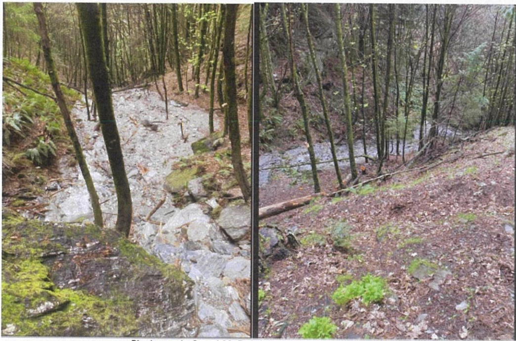
Photographs 9 and 10. Debris in Area 2 - Reavers Creek.
