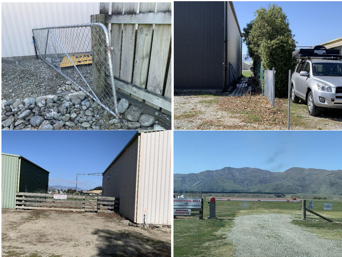
(clockwise from top left; unsecured gate, no fencing between hangars, inadequate fencing, barrier arm pedestrians and animals can get under or around)
