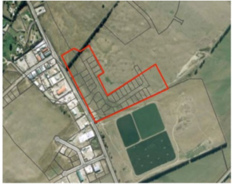
Aerial photo of subject site showing approximate area of re-zoning request as it relates to Three Parks (red border).
