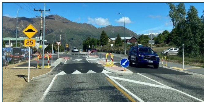
Figure 54: LCLR upgrade at Anderson Road Wānaka
