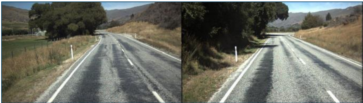
Figure 87: Examples of flushing on Cardrona Valley Road
