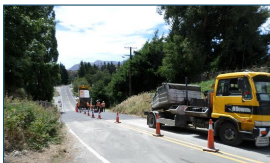
Figure 80: Sealed Pavement - Roadworks
