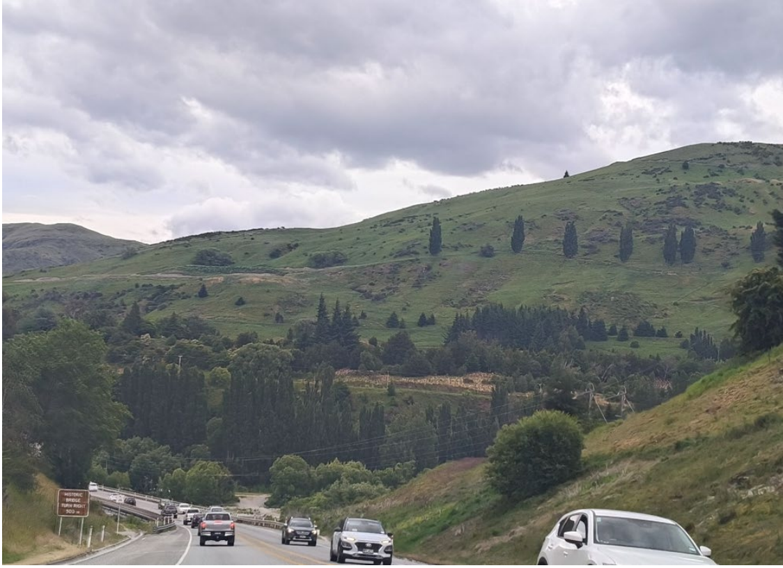
Figure 11. View of QRSZ from SH6
