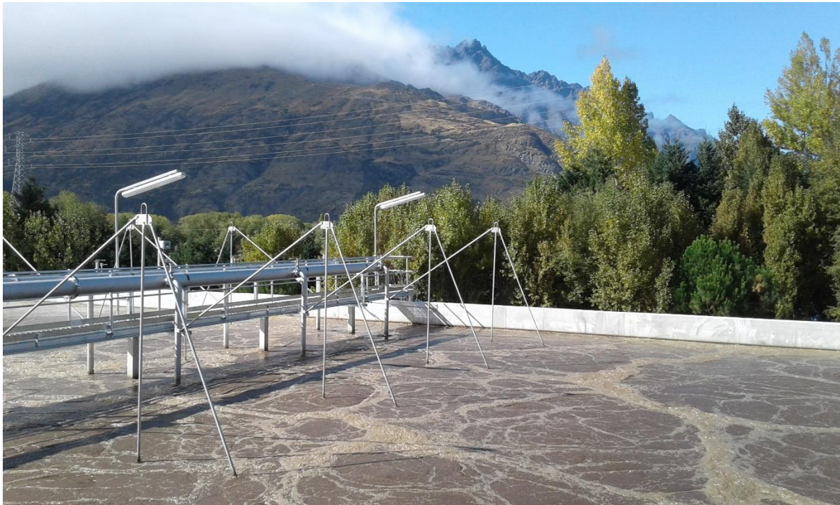
Figure 11: MLE Reactor aeration zones
