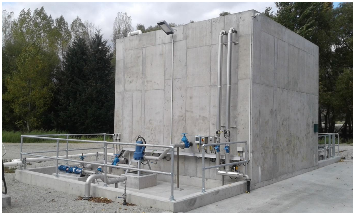
Figure 9 : Septage reception tank
