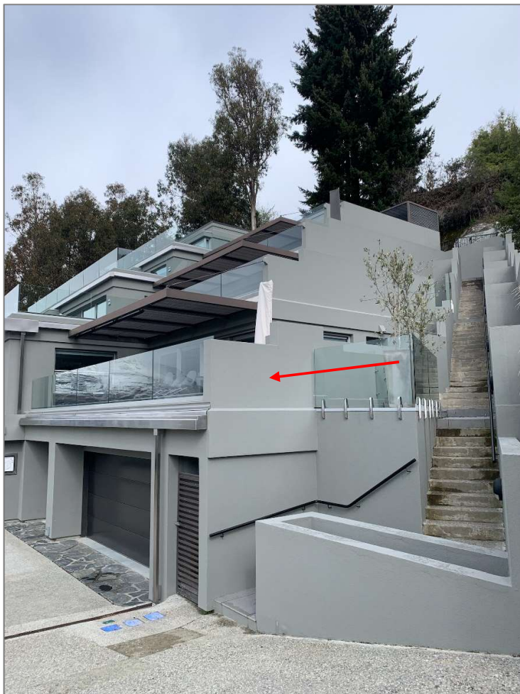
Figure 2: View from access showing solid screening on wall on north side of balcony (shown by red arrow).
