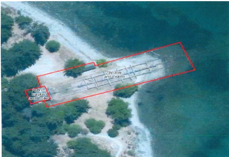
3a and 3b - Antrim Engine and Boiler, and Slipway and Cradle, Kelvin Peninsula. The Extent of Place is shown by the red outline
