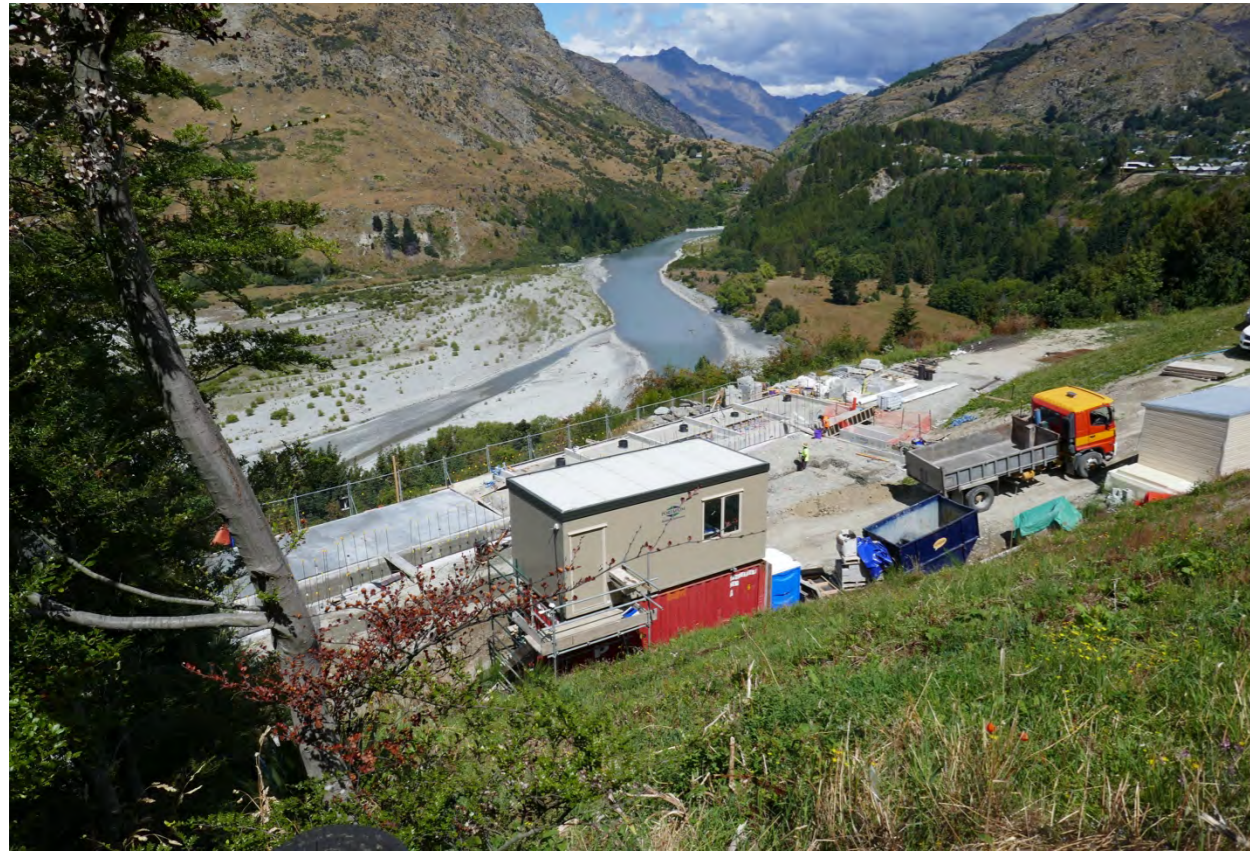
Photograph 8: View over Onsen Pools extension to Shotover River (photograph taken at 50mm lens equivalent on 22-02-19)
