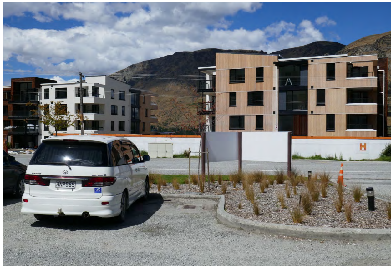
Photograph 6: Multistorey apartments within the zone (photograph taken at 50mm lens equivalent on 22-02-19)
