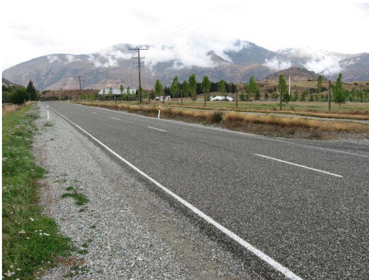
Photograph 4: McDonnell Road, Looking South at Existing Golf Course Entrance
