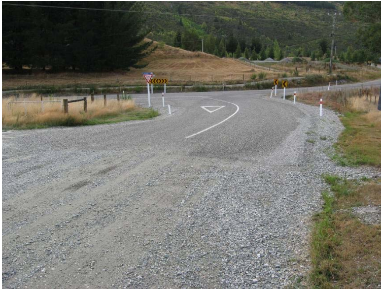
Photograph 7: Hogans Gully Road, Looking Towards Intersection with McDonnell Road
