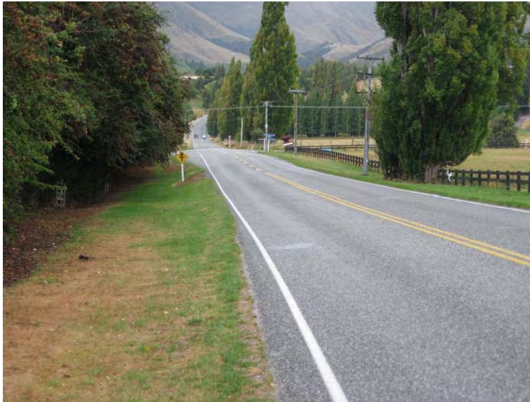
Photograph 1: Arrowtown-Lake Hayes Road, Looking North Past Hogans Gully Road
