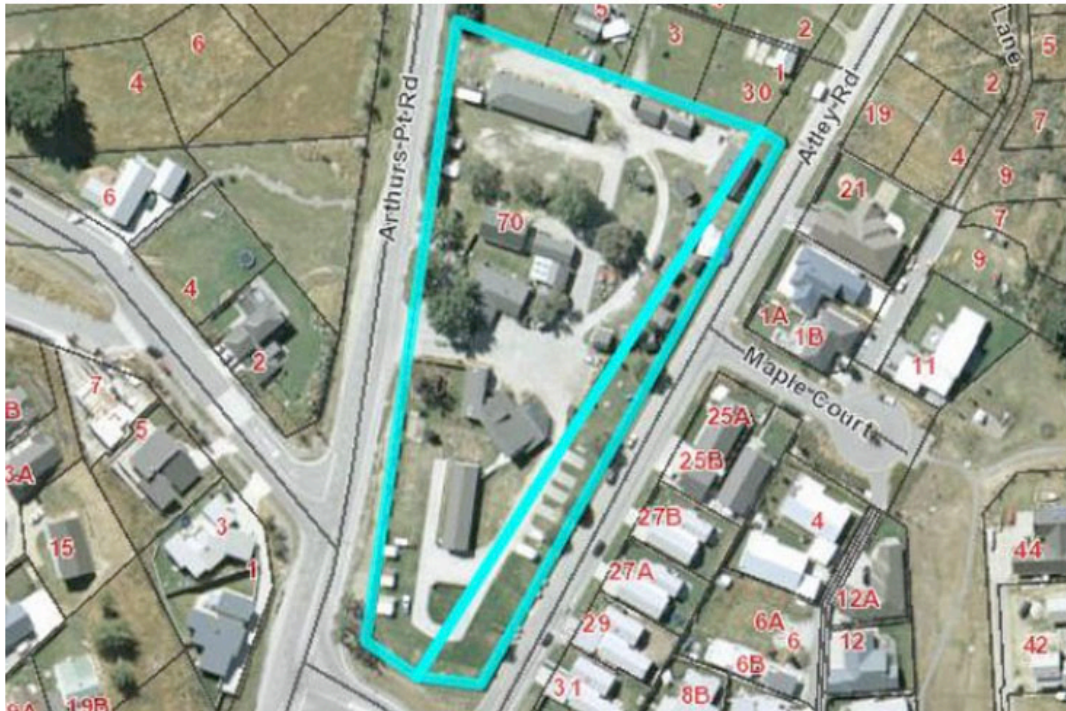
Figure 2-12 Aerial Photograph showing land subject to the submission outlined in blue
