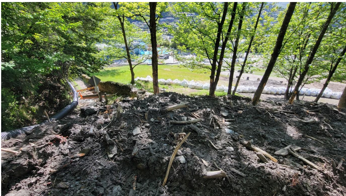
Lots of material still to be cleared from above the cemetery (above)
