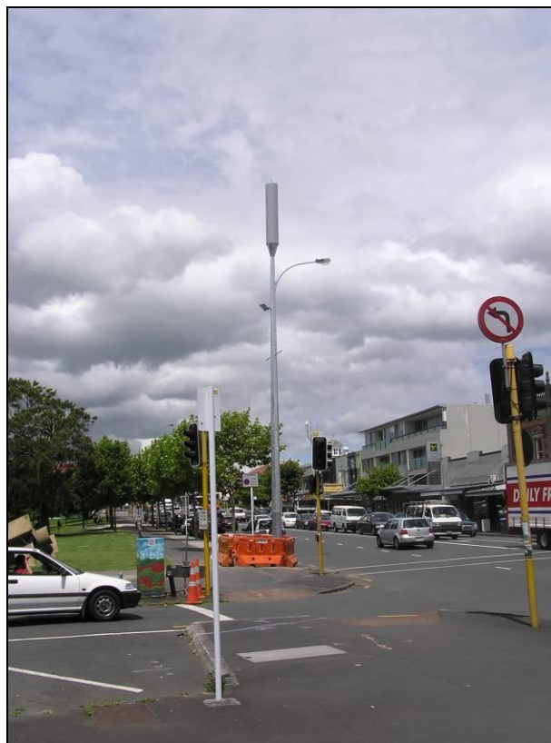
Figure 2: Typical Spark light pole on Ponsonby Road, Auckland (example is 15m high)
