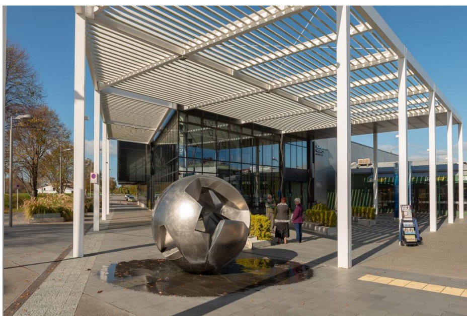
Kaipoi Library, Ruataniwha Centre, Waimakariri District Council
