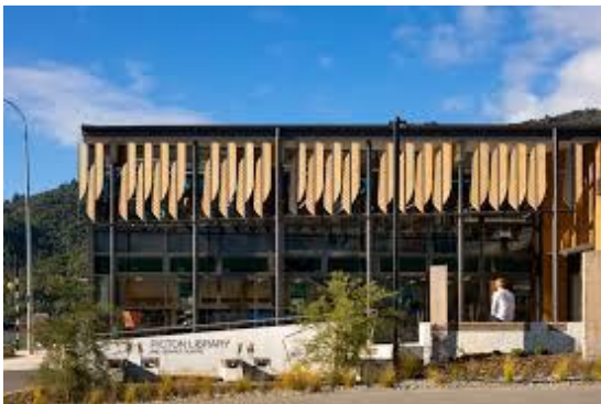
Picton Library © Athfield Architects
