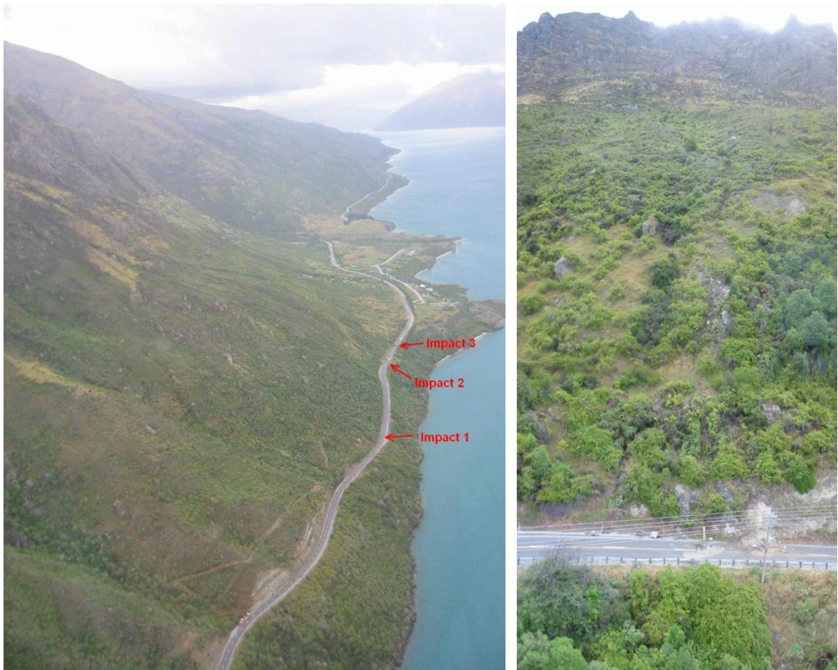
Illustration 3 - Recent Rockfall impacts on SH6 (Drift Bay development visible in the background)
