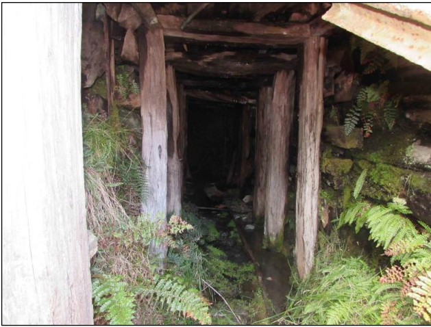
Figure 5-20. Timbered adit at Gollop No. 1 (??)
