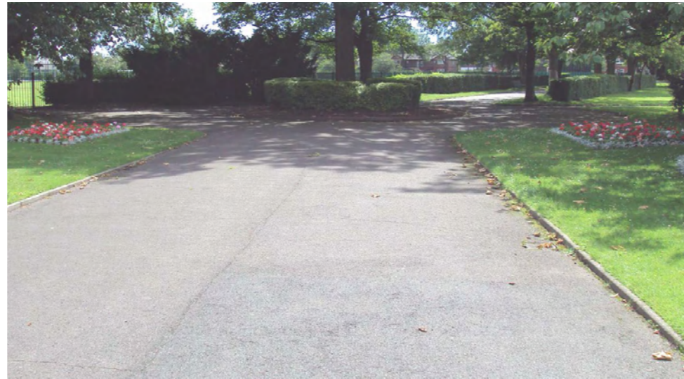
Sealed vehicle access roads / carparking
