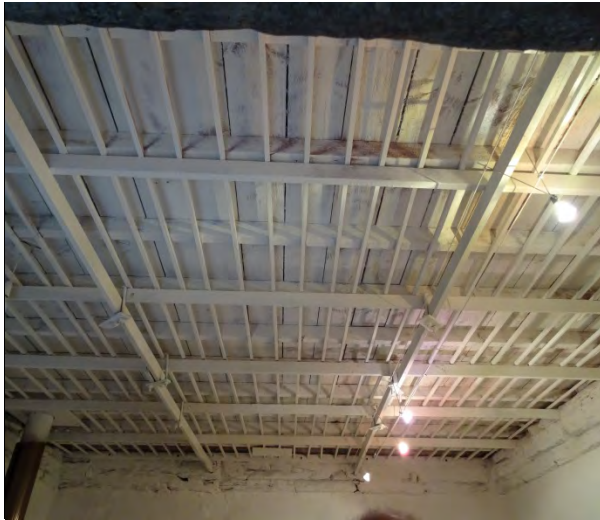
Sprung floor of oast house, December 2013
