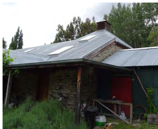
View of south side, December 2013
