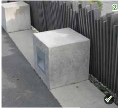
Recessed bollard lighting
