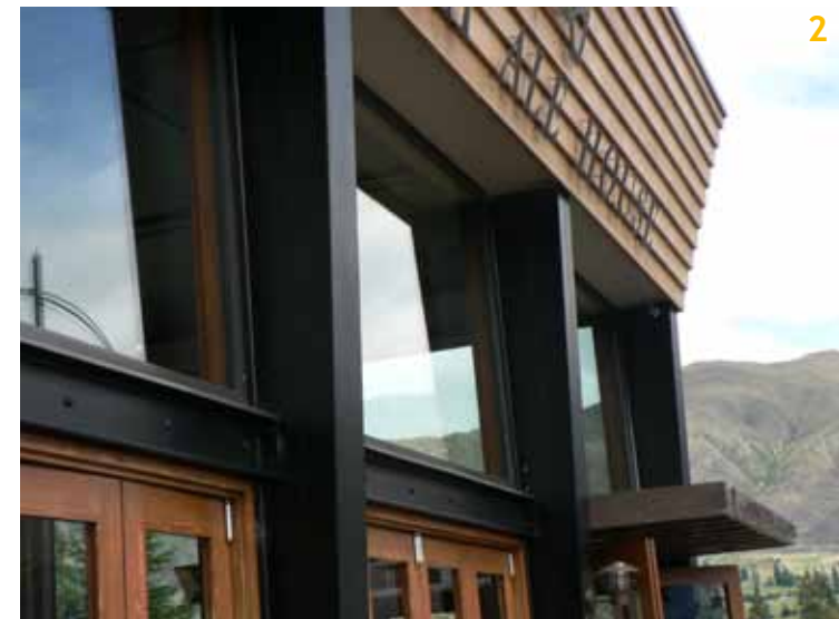
Steel columns & lintels
