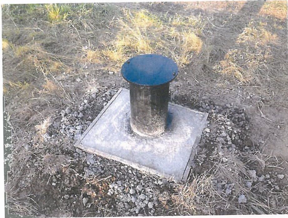
Figure 3: Example of finished bore
