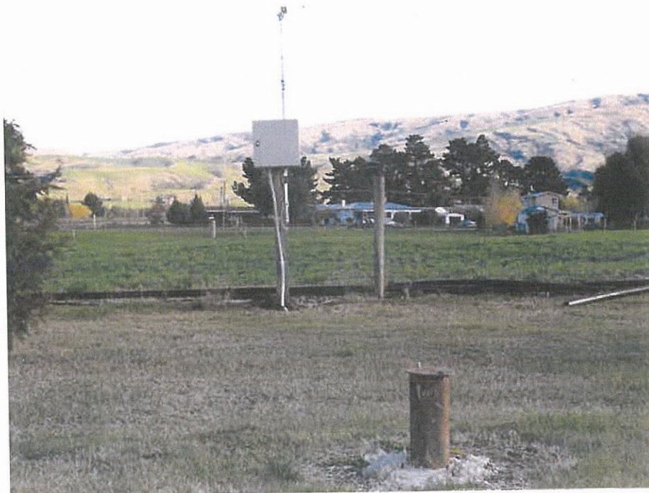
Figure 4: Example of finished bore and telemetry system.
