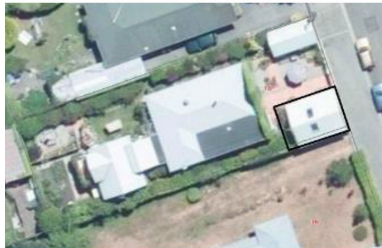
58 - Stone Building - 17 Brisbane Street, Queenstown. The Extent of Place is shown by the black outline.
