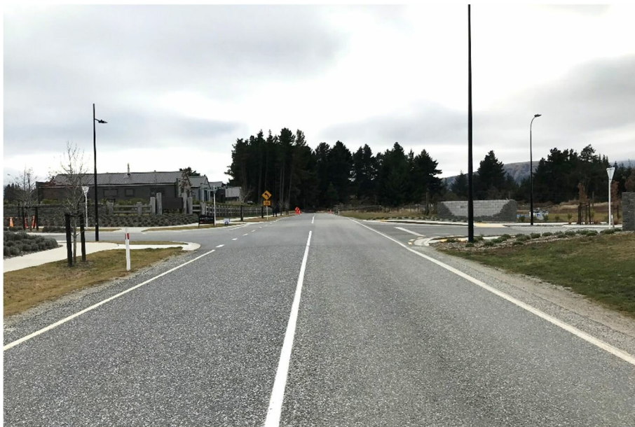
Photograph 3: Outlet Drive Looking North, Northlake Drive on Left
