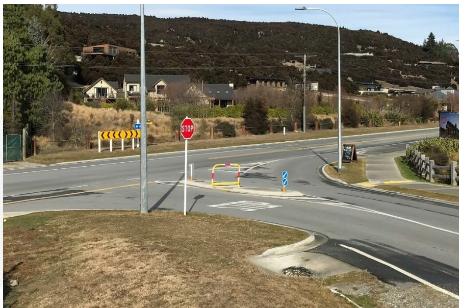
Photograph 4: Aubrey Road / Outlet Road Intersection
