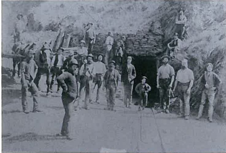
Figure 13. Tipperary Gold Mine, Macetown. c.1880s. Lakes District Museum Collection EP 3209
