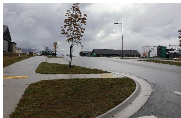
Photo N: Riverslea Road - kerb buildout at intersections
