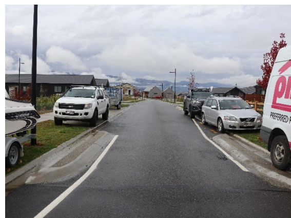
Photo H: Lammermoor Street Road localised narrowing
