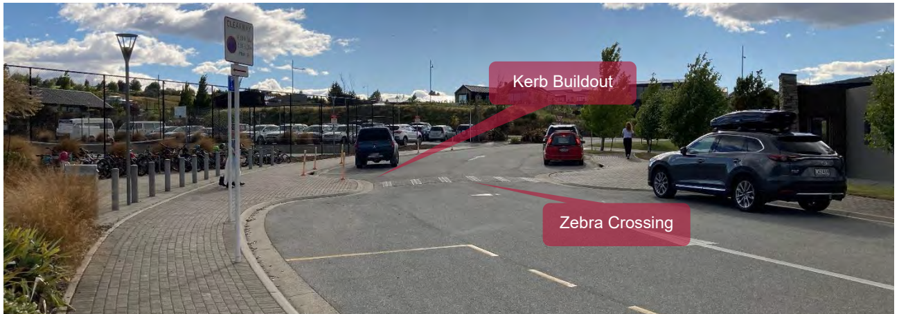
Figure 4.26 Pick up and Drop off Zone, zebra crossing and kerb build out
