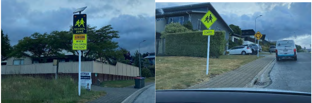
Figure 4.30 School sign and electronic variable children crossing sign.
