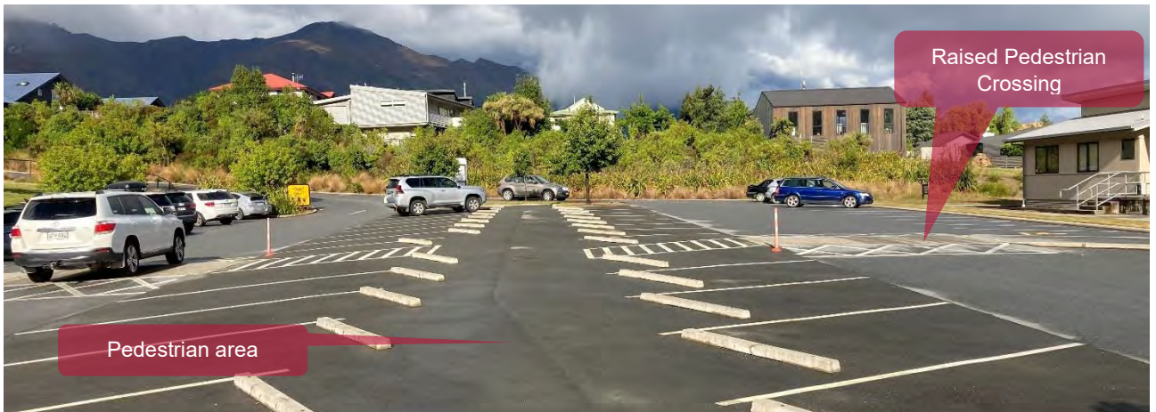
Figure 4.35 Totara Terrace Car Park
