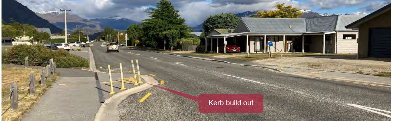
Figure 4.24 Kerb build out with tactiles
