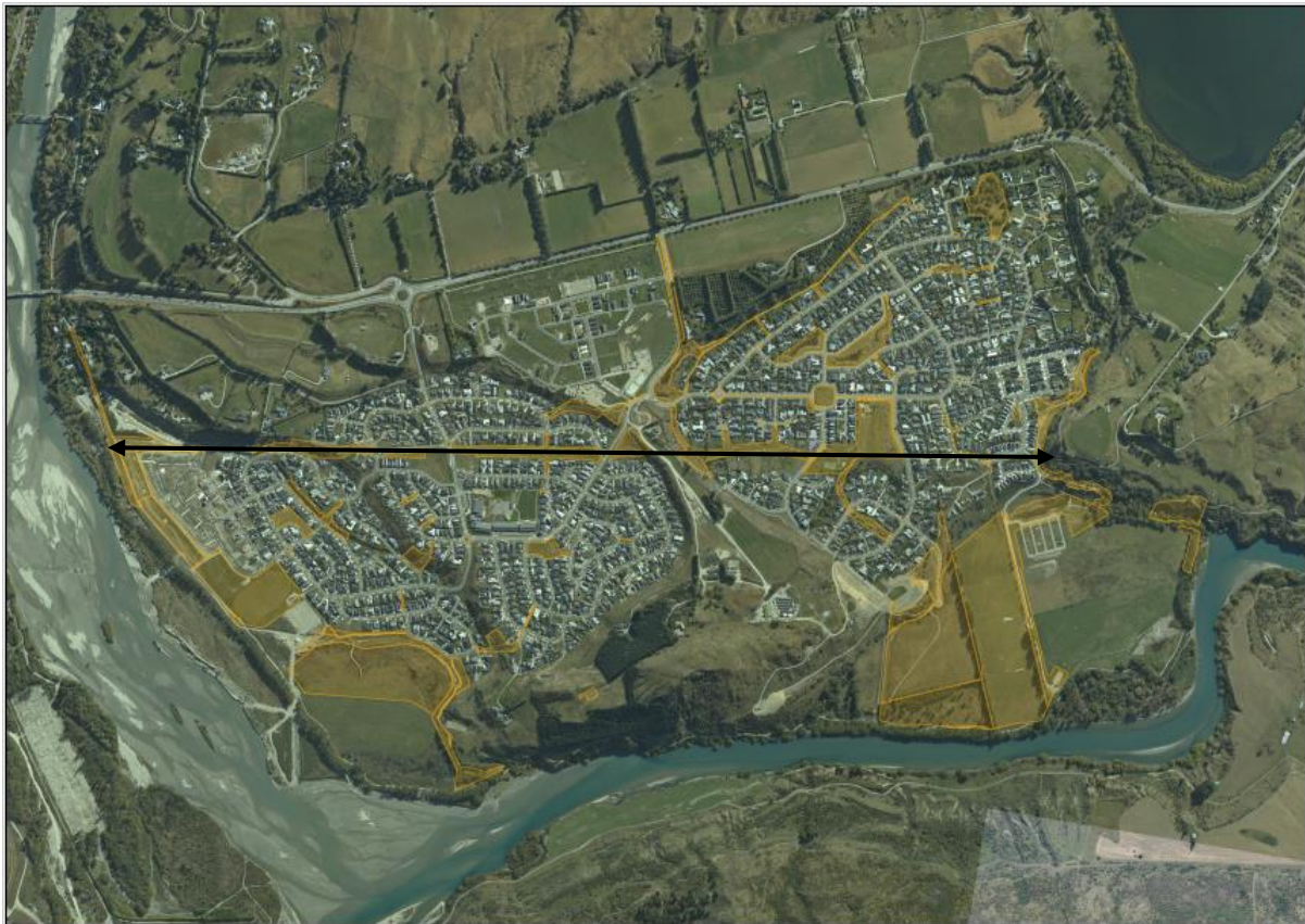
Image 2 High voltage transmission power line ~2.7km
