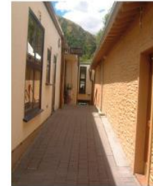
Uninteresting pedestrian link with poor detailing.
