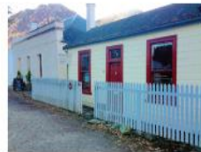
Good example of Picket fencing outside Miner's Cottage, Buckingham Street.
