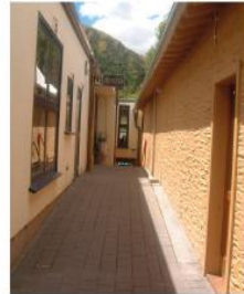
Uninteresting pedestrian link with poor detailing.
