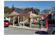
Open Space area to the north west side of Post Office, which is now integrated with the Post Office Precinct development to the rear.
