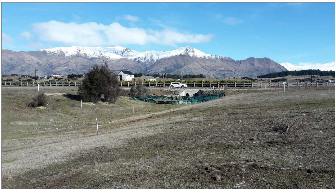
Figure 2: Outlet Road overland flow path and sediment fence (Twin culverts indicate flow potential from upstream catchment)
