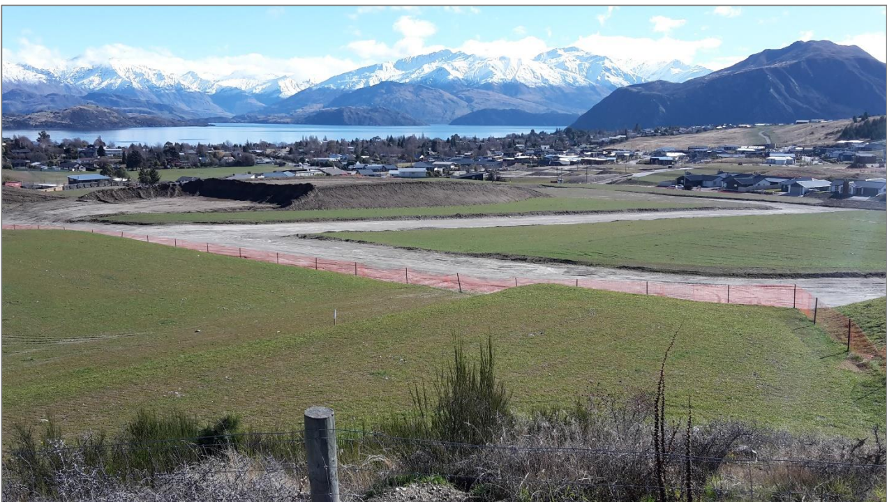
Figure 5: Unstabilised topsoil stockpile
