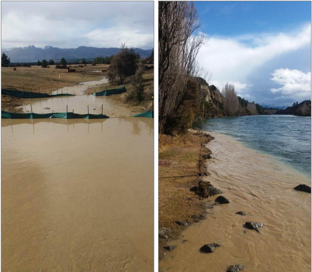
Figure 3: Outlet Road overland flow path and silt fence failure with sediment discharge to the Clutha River
