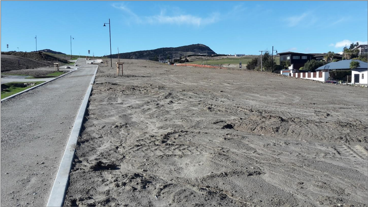
Figure 4: Unstabilised slope with rill erosion. Note planted trees indicating works are complete with finished contours
