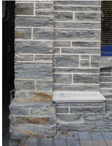
Council Chambers, 50 Stanley Street (tuck-pointing)
