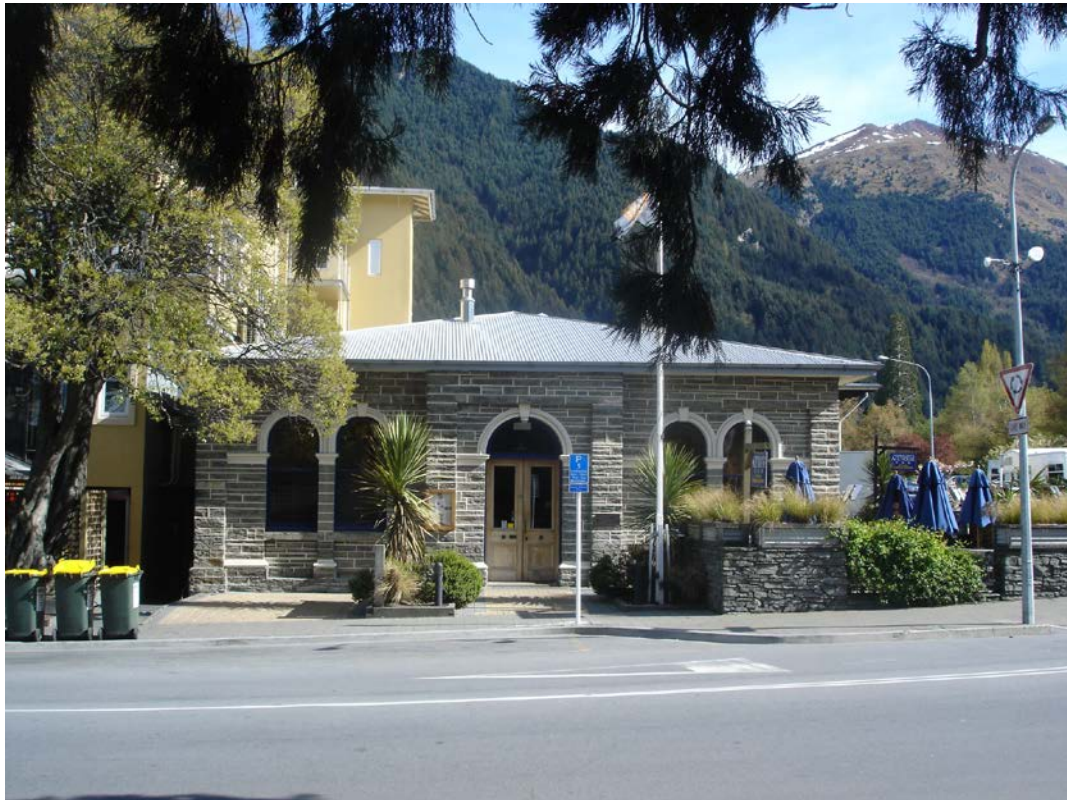
Old Council Chambers, Ballarat Street.
