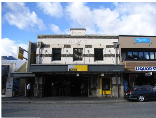
ASB Building, 24 Camp Street
