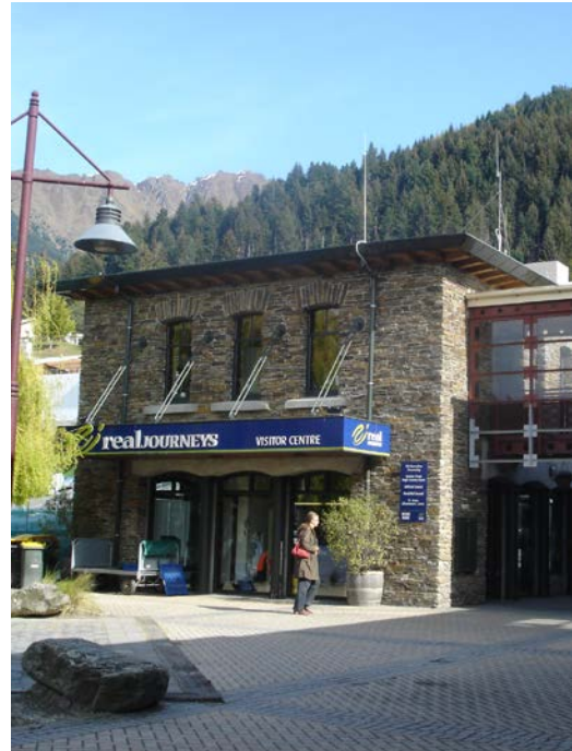
Steamer Wharf, 88 Beach Street
