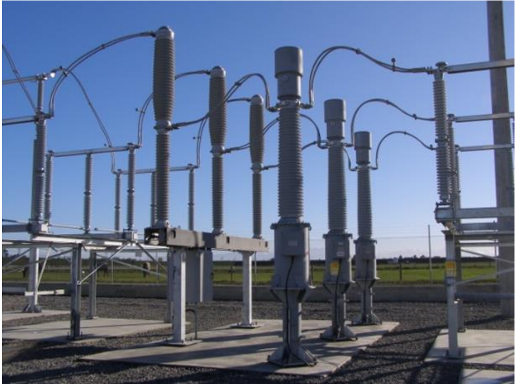
Photo 1: Circuit breaker, Current Transformer, Disconnect
