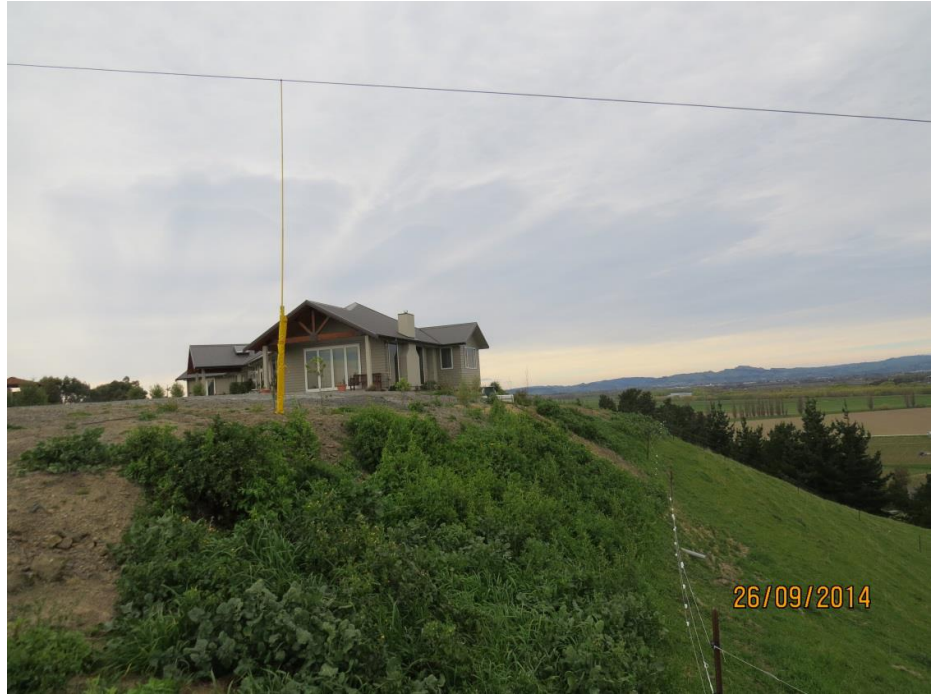
Photo 5: Ground clearance violations in Hastings
