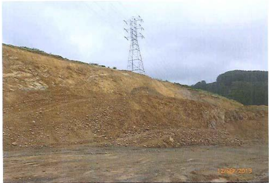
Photo 2: Earthworks in Porirua, Wellington
