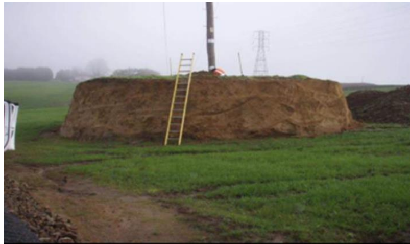
Photo 3: Excavations compliant with NZECP34 around base of pole
