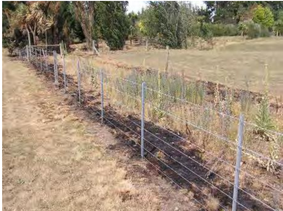
Photo 1: Fence and surrounding area affected by Earth Potential Rise, near Geraldine, South Canterbury
