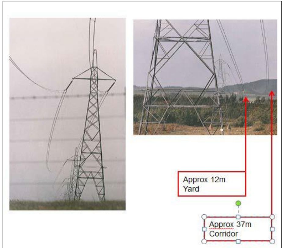
Photo 1: Conductor swing in high wind
