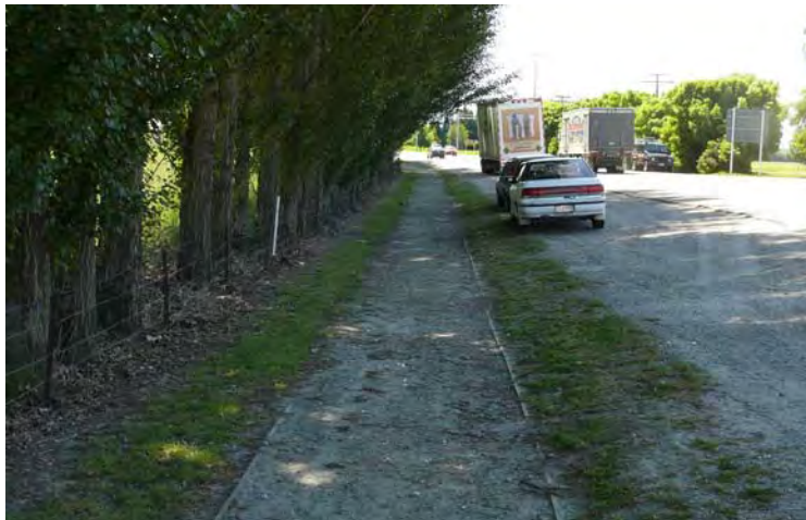
Pedestrian path along subject site frontage
