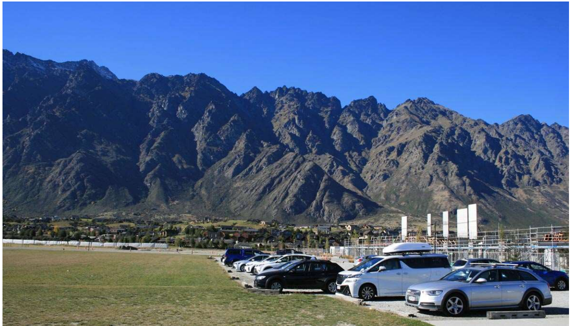
Figure H – View looking east along McAdam Drive with the Remarkables in the background, towering over the existing residential of Jacks Point beyond the village. The development to the right is a mixed use three and four level building under construction (M-7).
