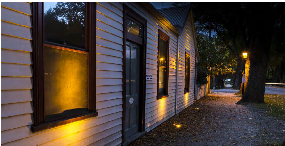
Completed lighting on Miners’ Cottages, April 2018
