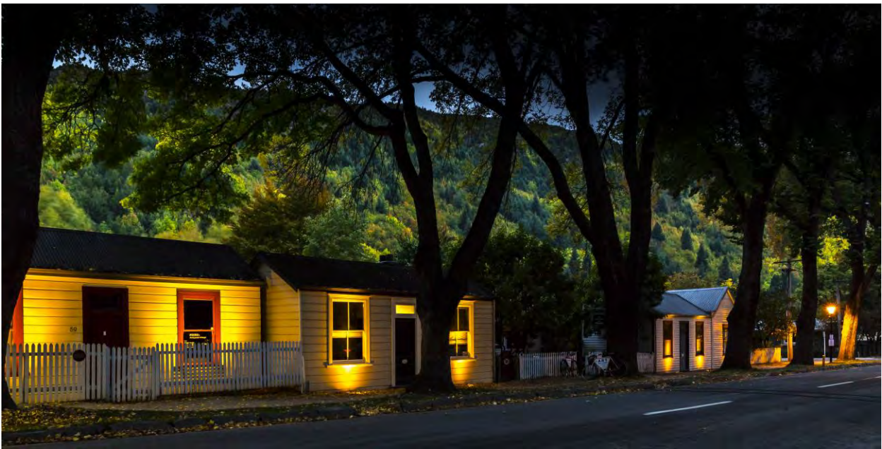
Completed lighting on Miners' Cottages, April 2018
