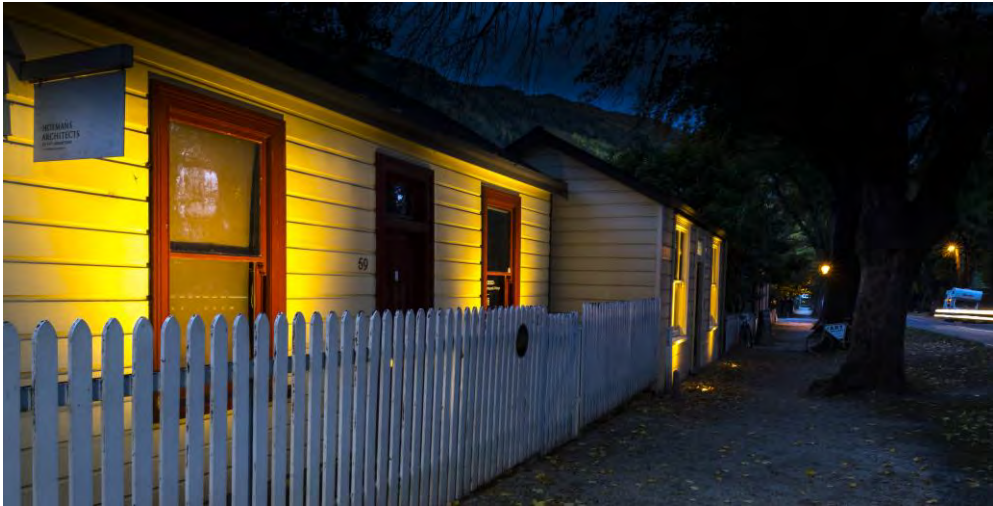
Completed lighting on Miners' Cottages, April 2018
