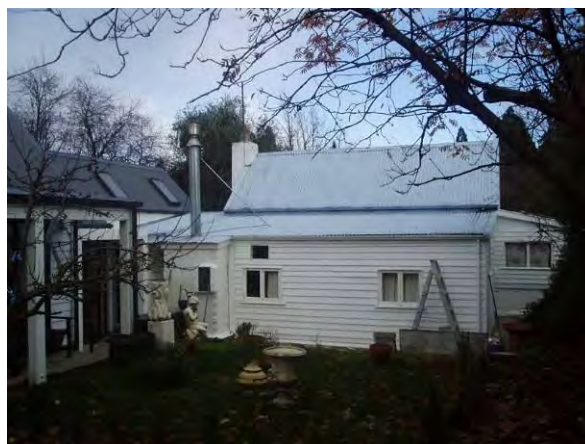
Rear of cottage, addition on left
