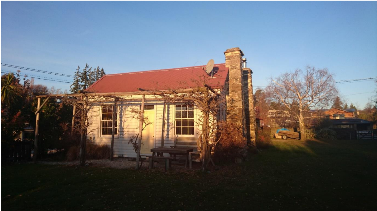
Photo 3 North elevation – Origin Consultants 28 June 2019
