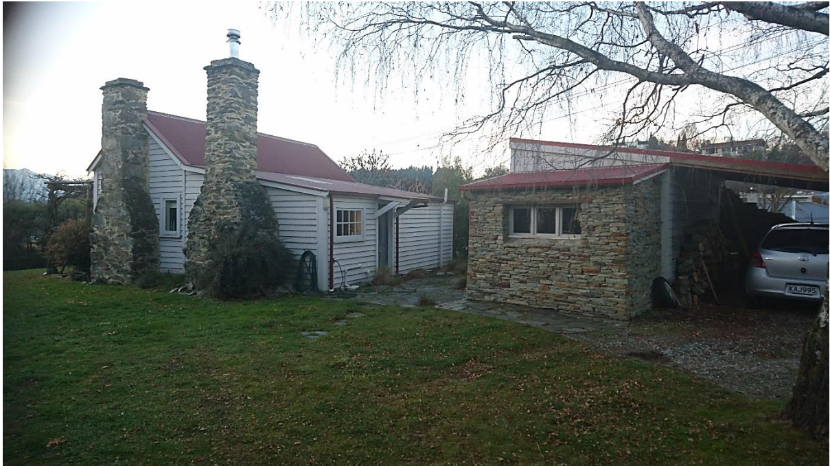
Photo 5 West and south elevations and modern outbuilding/carport – Origin Consultants 28 June 2019
