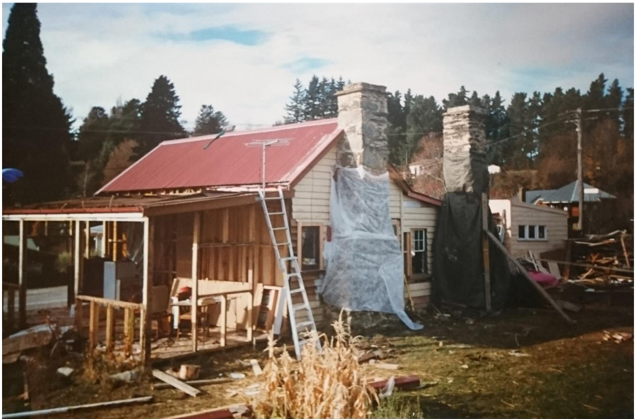
Photo 6 Refurbishment c. 1994 – photo supplied by present owners
