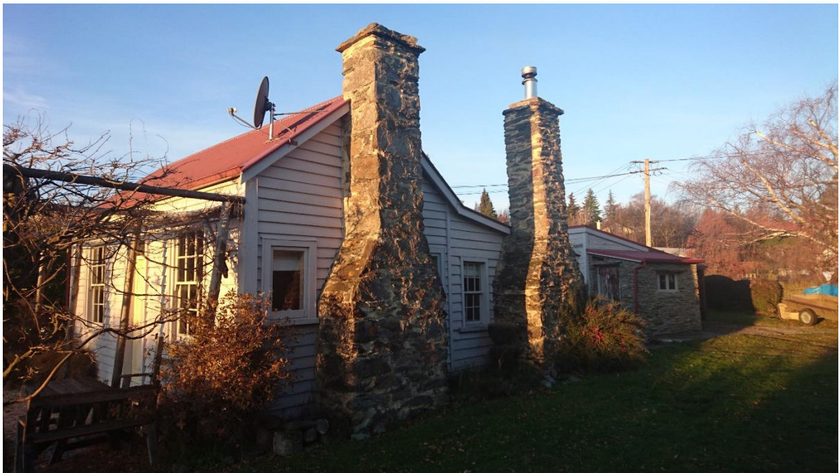
Photo 4 West elevation – Origin Consultants 28 June 2019
