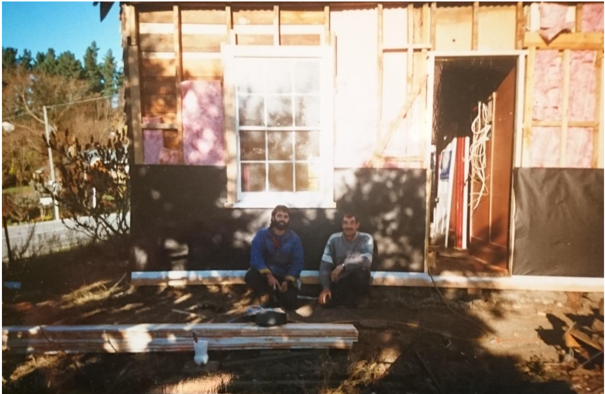
Photo 7 Refurbishment (north elevation) c. 1994 – photo supplied by present owners
