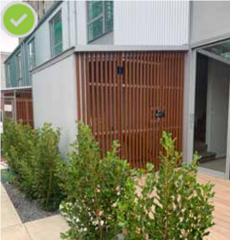
Each unit is provided with screened storage facility
