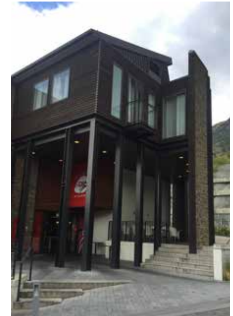
First floor residential units provide passive surveillance over public spaces at all hours.
