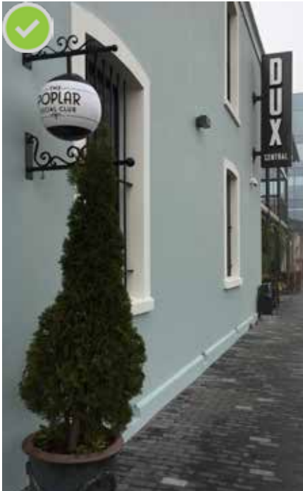
Signs can be integrated into lighting and other elements so as not to appear an add-on
