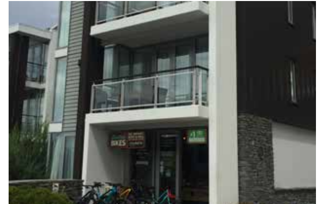
Small ground floor units provide space for a diverse range of businesses.
