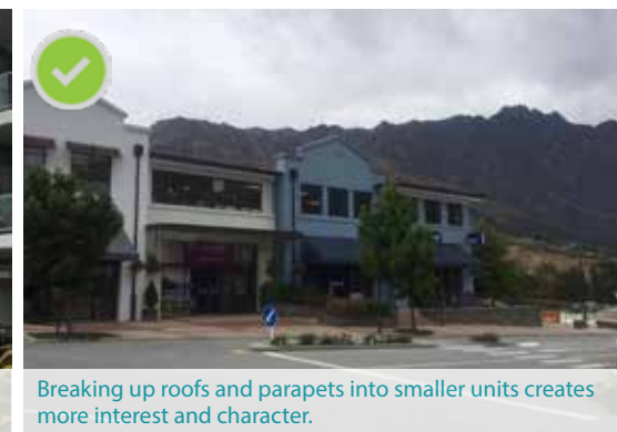
Modulation of roof forms helps to reduce the visual mass and monotony of a development
